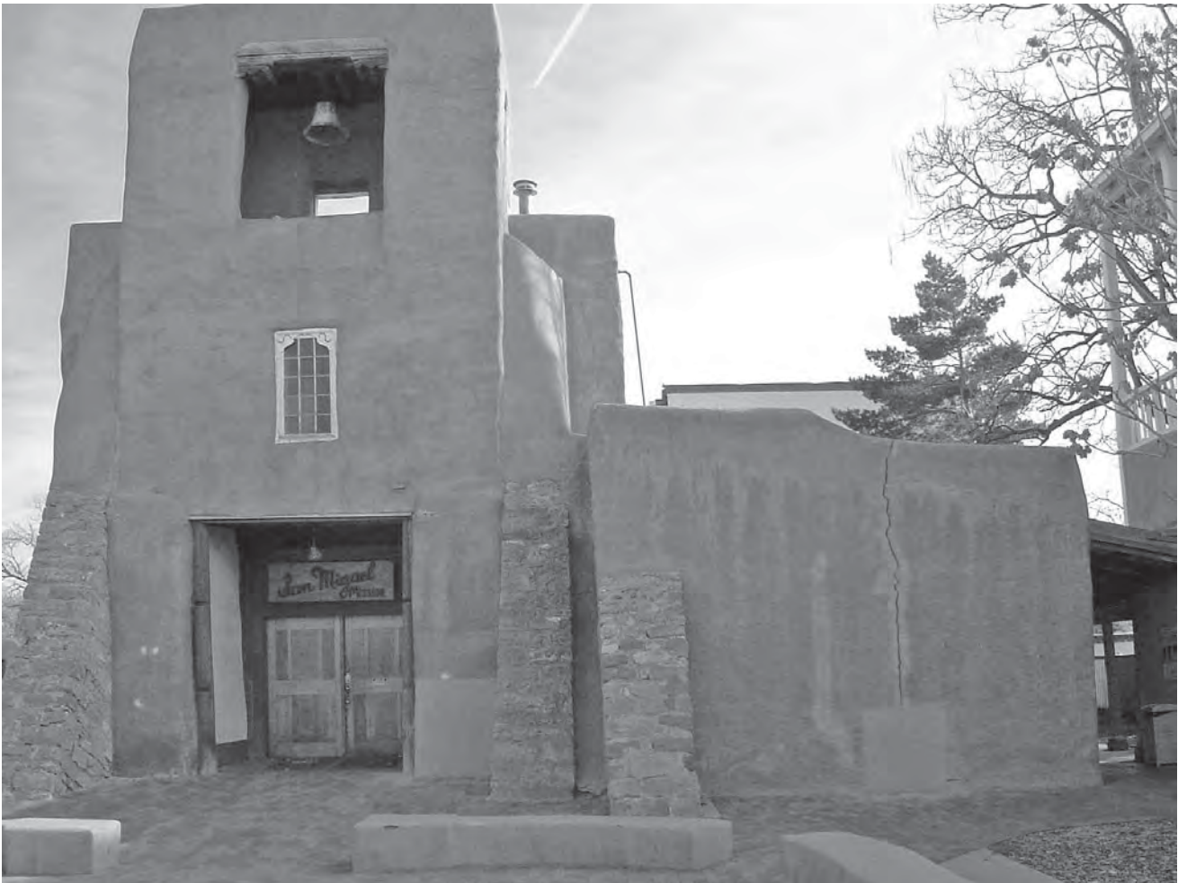
San Miguel Catholic Church, Santa Fe, New Mexico. Built about 1610, it is the oldest church structure in the United States. (J. Gordon Melton)
