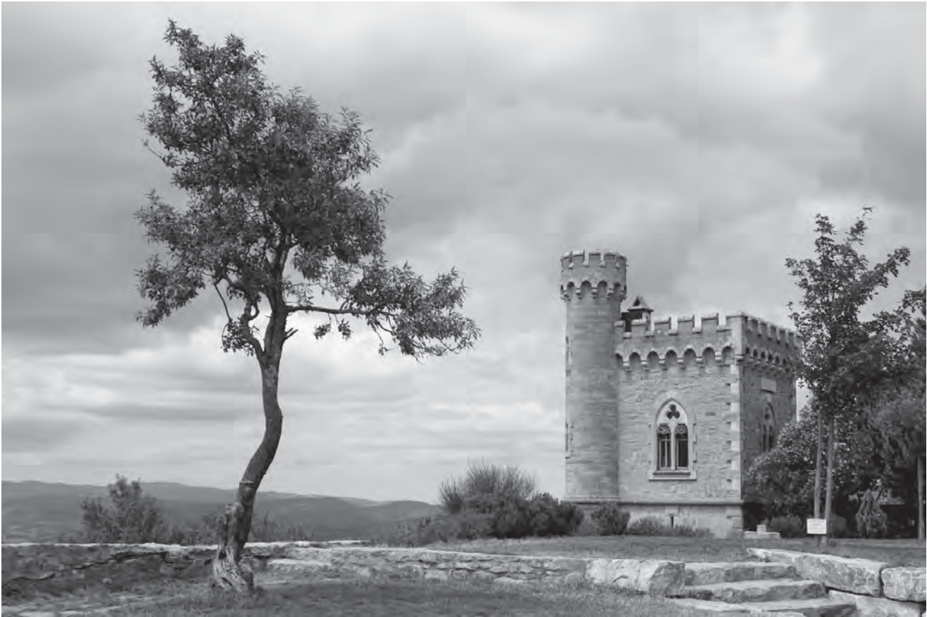
The gothic “Tower of Magdala,” built by Berenger Saunière, the eccentric parish priest of Rennes-le-Château, a small village in southwest France. (Andreas Stecher/StockphotoPro)
